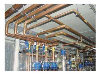
Thanks to its viscosity even at low temperatures the copper tube is not only perfectly suitable for the installation of technical gases but also less expensive than stainless steel. The tubes are hard soldered and connected using silver solder.
